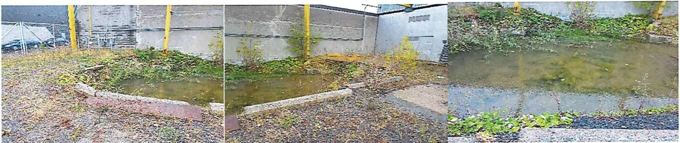
Arrived at the site approximately 10:30am on November 5, 2018 to meet with the Montreal operations operator on unit #1128. At the time of arrival, the Battlefield equipment was being delivered and everyone was briefed on the proposed scope of work. Once completed, the operator began to remove the first load of water from the back of the excavation. 2 ½ loads of water were ultimately removed from the excavation.
