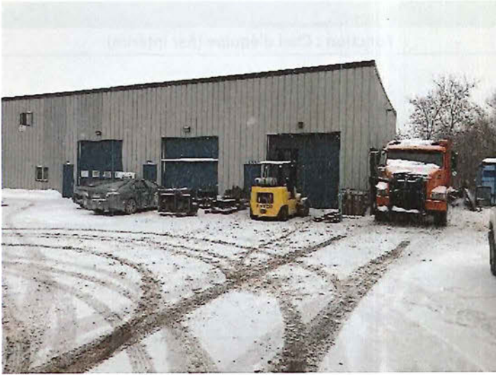
IMG_0153.jpg Photo no. 1
