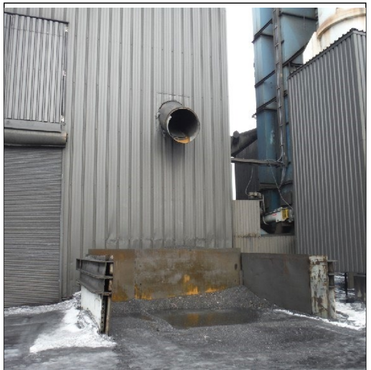
DSCF1831.JPG Photo 12: Chute
