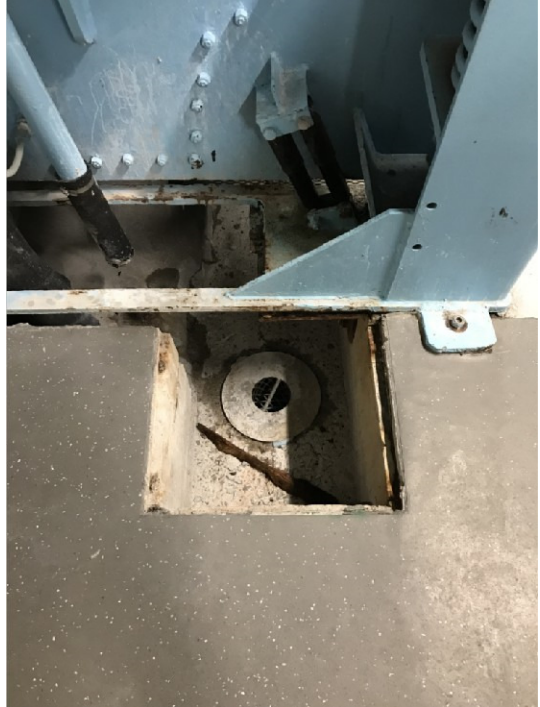
IMG_1157.JPG Image 5. Drain
